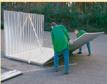
1. Install the side walls
