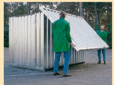
4. Put on the roof – finished!
