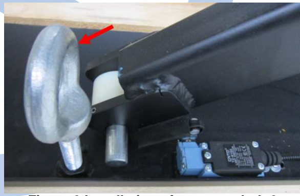
Figure 9 Installation of transport bolt 2
