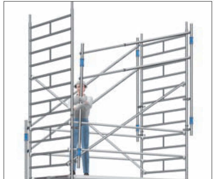
Fig. 5: Upward movement of the advance guardrail system
