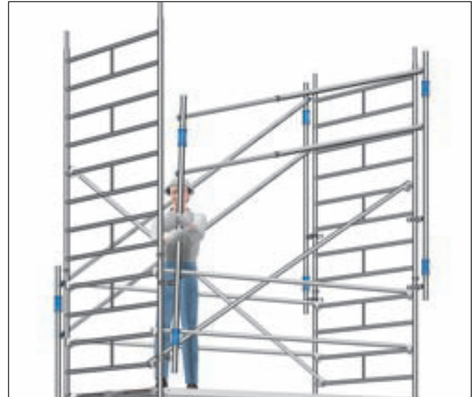
Fig. 5: Upward movement of the advance guardrail system
