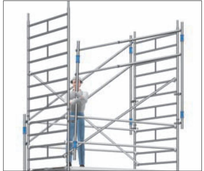
Fig. 5: Upward movement of the advance guardrail system
